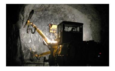
Initially a smaller  $5 \times 6m$  relief tunnel was conventionally blasted in the top middle section of the larger tunnel excavation.
